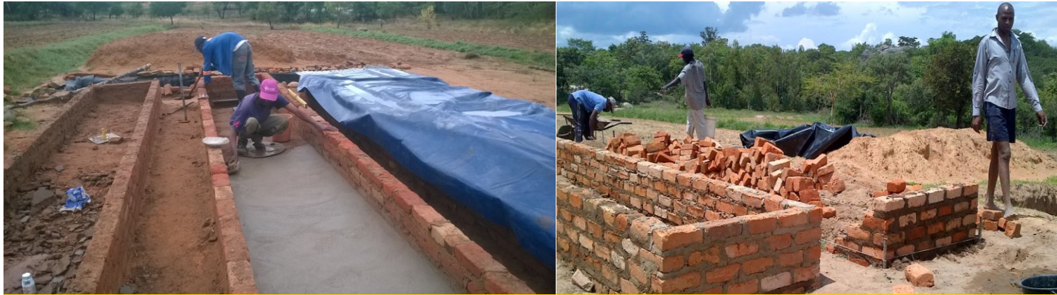
Clive and his Shift Organic Technologies team building and setting up structures to implement the VA System project at a much larger scale in his Svosve communal lands in Wedza.
